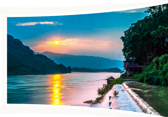
● 东风堰 / Dongfeng Weir
